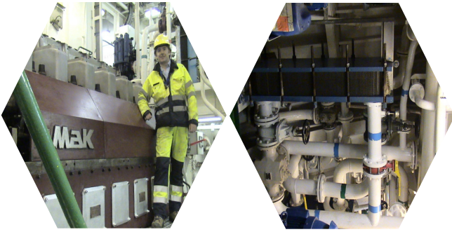
ENGINE ROOM SURVEY
